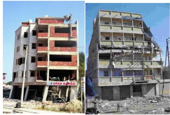
Fig. 3: (a) Ground soft storey failure, Fig 3(b) Intermediate soft storey failure
