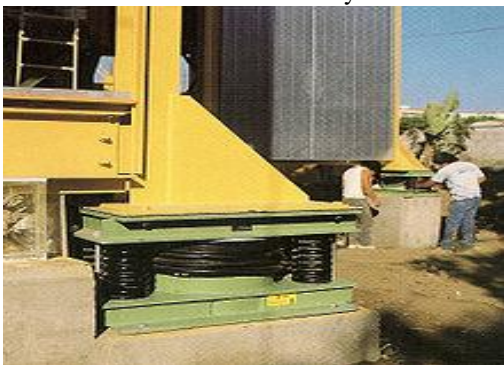
Fig. 7: Spring Base Isolator [17]
