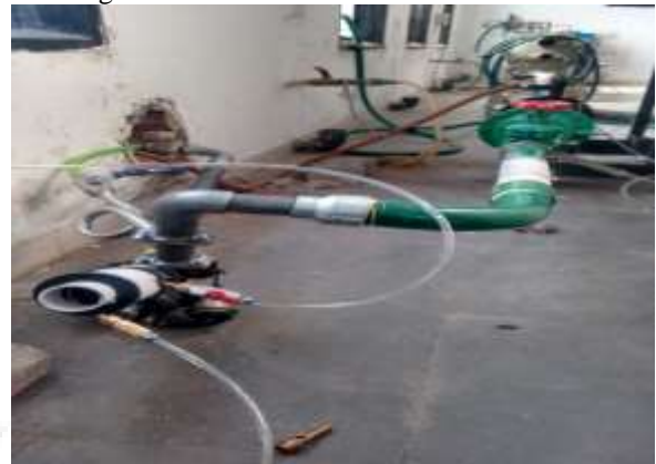
Fig. 2: Turbocharger with Wastegate Valve And Intercooler Installed At Exhaust Line
