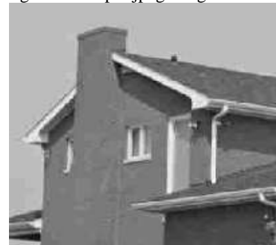
Fig. 3: The compressed jpeg image of house.
