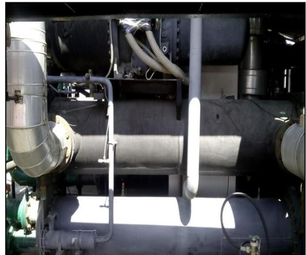
Fig. 3: Water Cooled Screw Chiller, Single Circuit Type (225TR/163KW).
