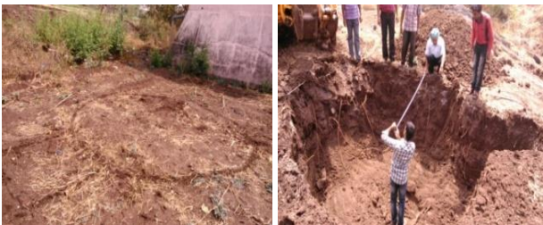
Fig. 3: Plant layout and Excavation works
