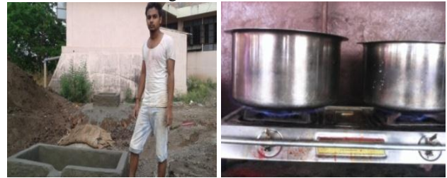
Fig. 5: Completed biogas plant and flame from burner
