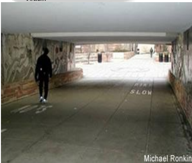
Fig. 1: Under Pedestrian Tunnel
