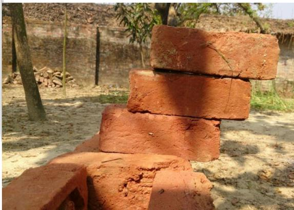
Fig. 4: Demonstration of Brick Corbel
