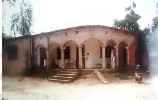
Fig. 1: Unplastered Work of ‘KAILASH KUTIR’ Built By Using Semi-Elliptical Brick Arches
