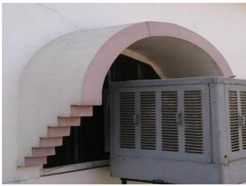
Fig. 3: Demonstration of Use of Extended Brick Arch over the Window Opening In the Exterior
