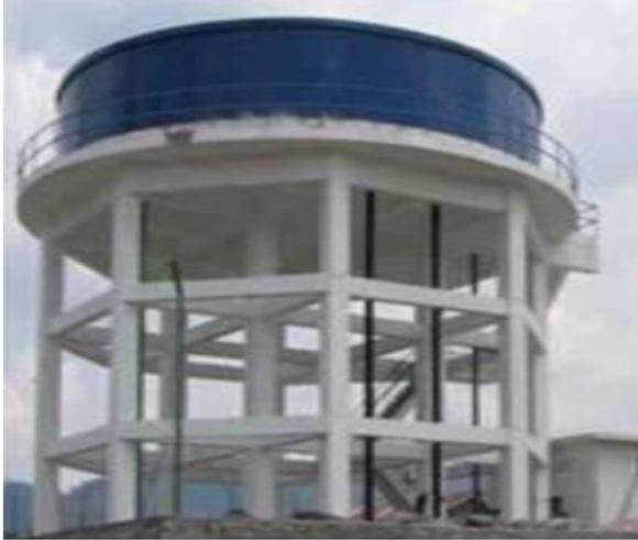
Fig. 1: Elevated Circular Liquid Storage Tank with Columns Rigid at Top and Fixed at Footings
