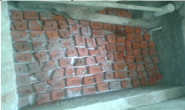
Fig. 3: Laying of brick bats
