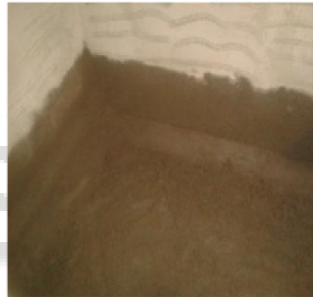
Fig. 4: Cementing after brick bates lying
