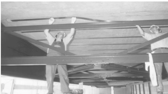
Fig 2: Application of prefabricated strips
