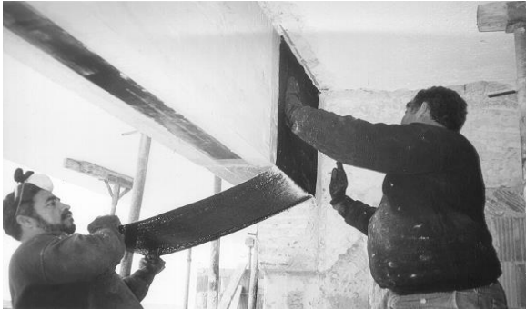
Fig. 1 : Wet lay-up of CFRP sheets
