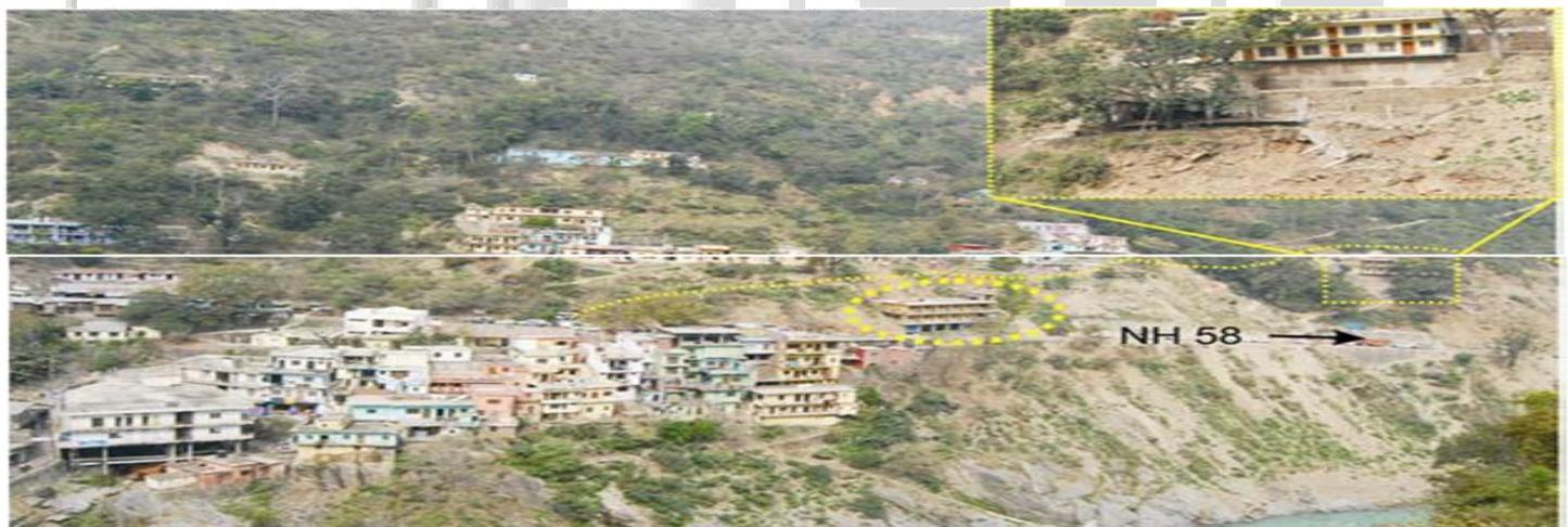
Fig-4- Slope failure and its geometry. Slope destabilization around Devprayag caused due to the widening of NH-58. Yellow Dotted line indicates the recent activation of the slope. House circled by yellow dots was partially buried under the Debris. (Inset) A house damaged due to disturbance of slope during road widening.
