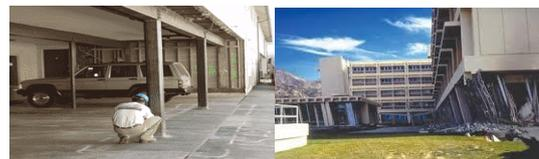
Fig. 3: Soft storey building failure during Bhuj Earthquake.
