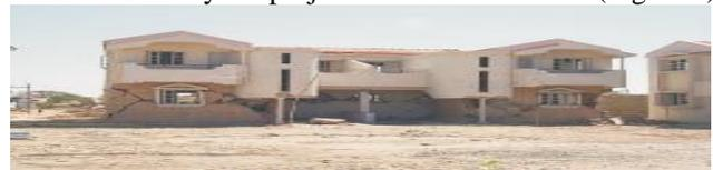
Fig. 4: Floating column building damage during Bhuj Earthquake
