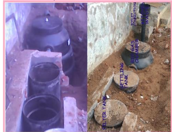
Fig. 5: Installations of toilet linked biogas plant at pratappura at domestic level
