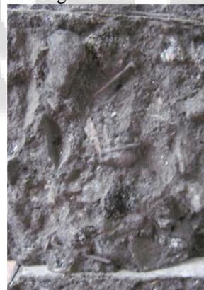
Fig. 9: Nail In Concrete
