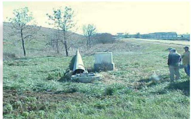
Fig. 1: Photograph of collapsed high mast tower
