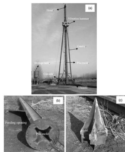
Fig. 1: Construction equipment: pile driving machine; (b) the mold of XCC pile; (c) valve pile shoe for the XCC pile.
