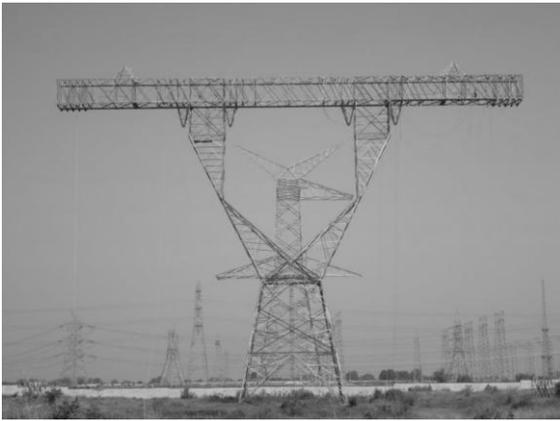
Fig. 2: 1200kV Tower Height: 55 m, Weight: 96 MT
