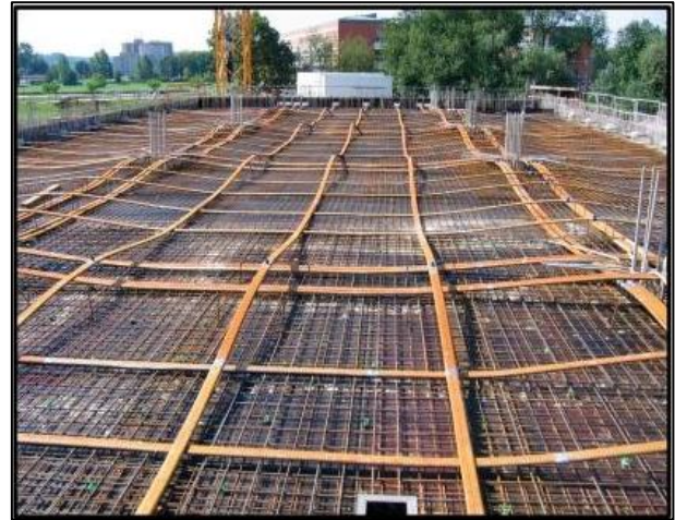
Fig. 8: Post tension slab system.
