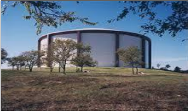
Fig. 1.3: Resting on ground level water tank
