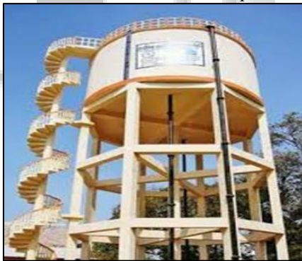
Fig. 1.4: Elevated water tank
