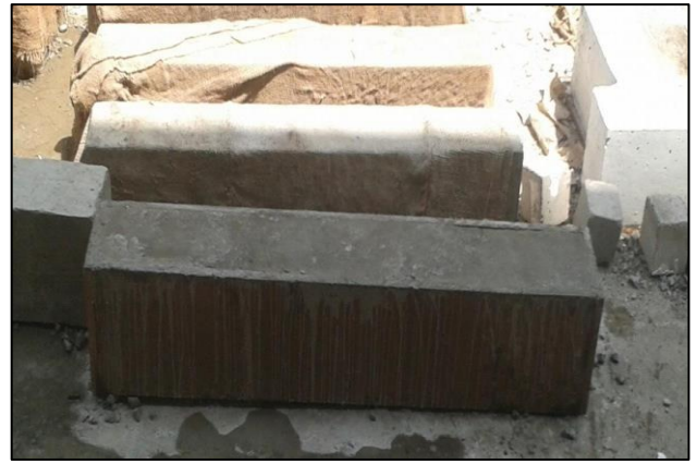
Fig. 12: Reinforced beams are cast
