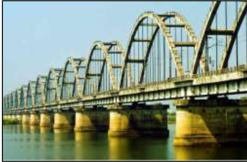
Fig. 5: Tied Arched bridges
