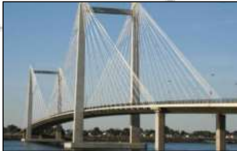
Fig. 7: Cable stand bridge
